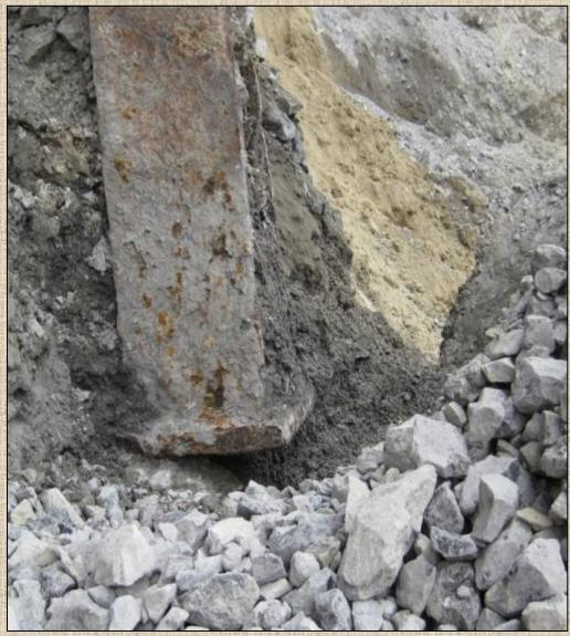
Foundation for walkway support is missing
