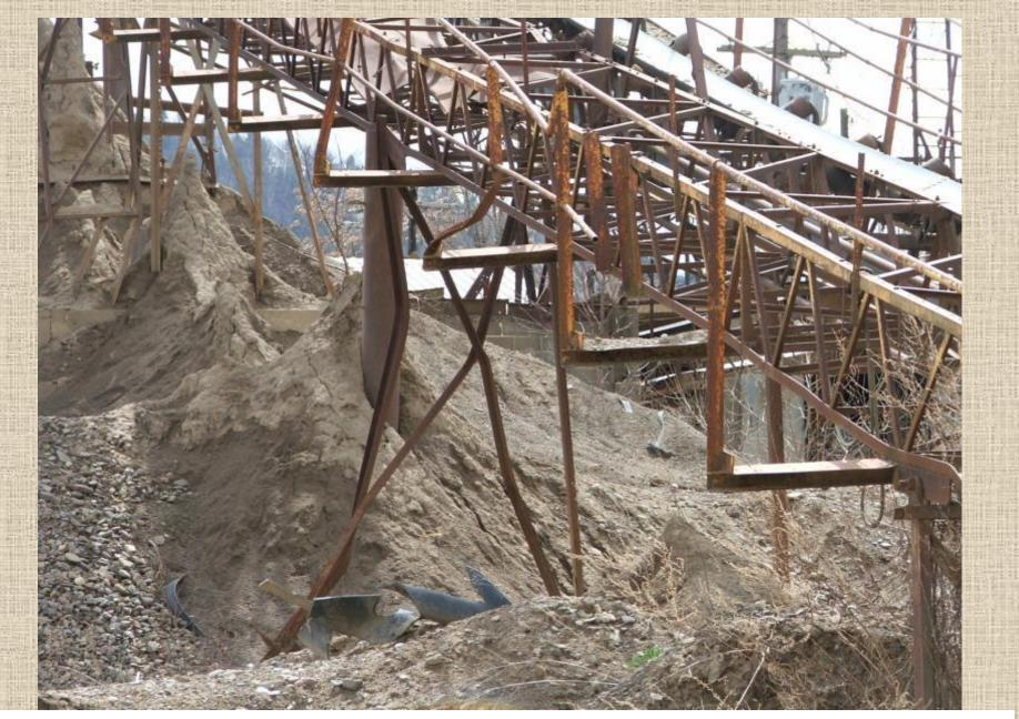
Impact damage to a conveyor bent and excessive material build, up
