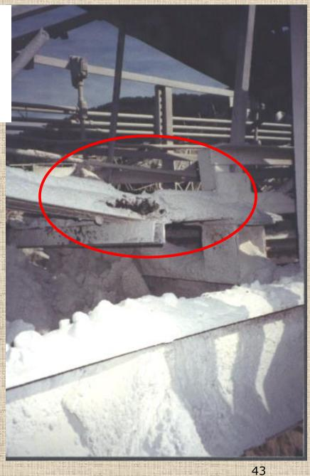
Deflected bottom chord that occurred because an added support post was not located at a joint
