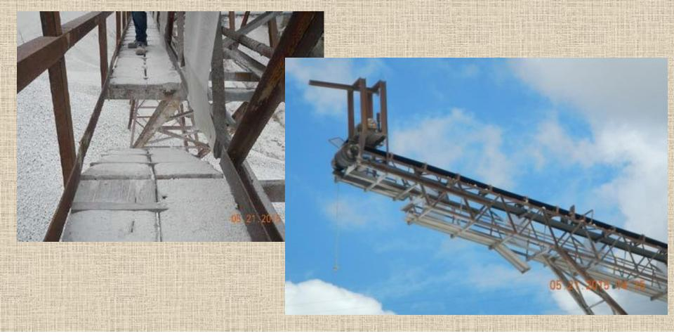
Near Miss - May, 2015 at a sand & gravel mine - An inspection party walked up the wood plank walkway to inspect the conveyor head pulley. As they started back down a section of the walkway unexpectedly dropped out from beneath the MSHA inspector leading the party. He escaped the 30 foot fall to the ground by holding onto the
