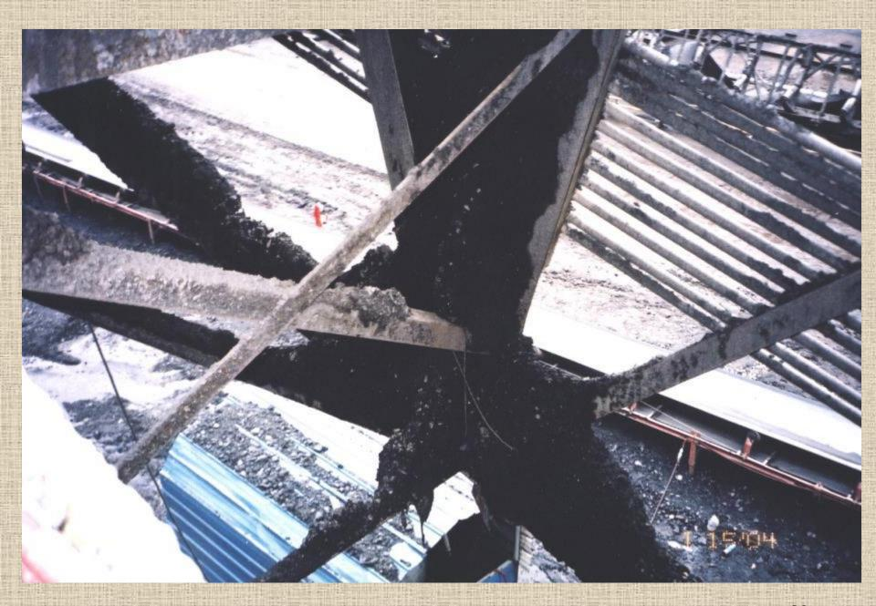
Accumulations on bottom chords and verticals add weight and may facilitate corrosion
