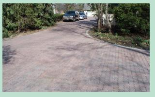
Porous Pavements are increasingly in demand as tools for managing storm water in an environmentally friendly way. They are an alternative to costly, bulky and land-intensive detention or retention ponds. In addition to the obvious environmental and land use benefits, installation of porous pavements can qualify for significant LEED® (Leadership in Energy and Environmental Design) points under the Green Building Rating System, developed by the United States Green Building Council (USGBC).
